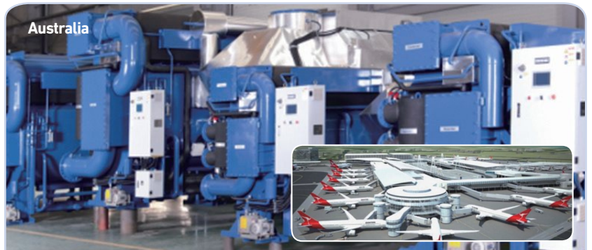
Qantas Trigeneneration at Sydney Airport CHP & HWAR-L 3,642usRT(12,805kW)
