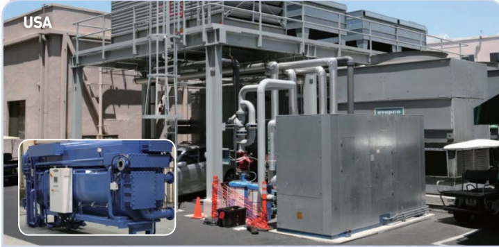
CBS Television City, with UTC HWR-L 50usRT(176kW)
