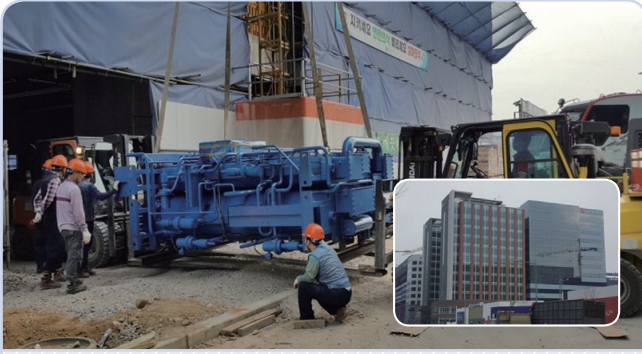
Hwaeom Building Munjeong-dong 2AB 270usRT(949kW)
