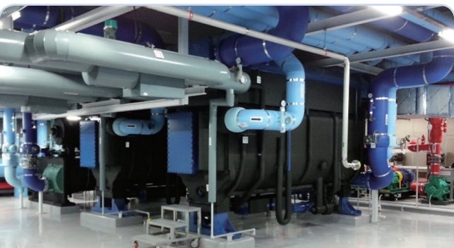
TOK HWAR-L 1,100usRT(3,868kW)
