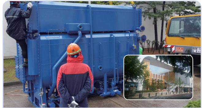
Yangcheon-gu Community Center 2AB 1,050usRT(3,692kW)
