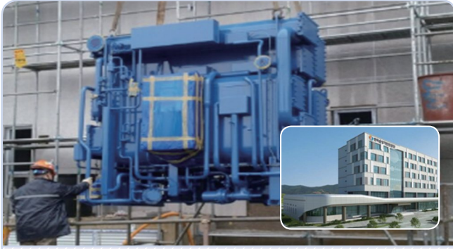
Korea Elevator Safety Agency 2AB 150usRT(527kW)
