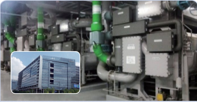
U-SPACE Pangyo 2AB 9 sets 6,295usRT(22,133kW)
