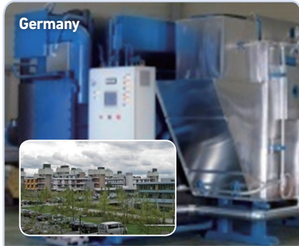
Giessen Hospital CHP 292usRT (1,027kW)
